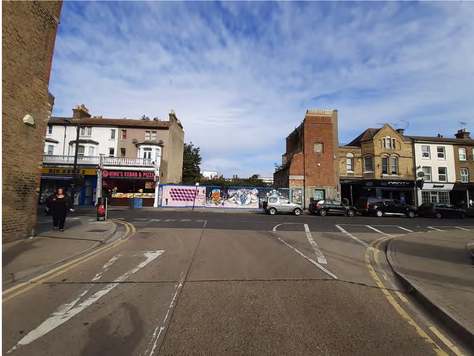
Alexandra Street frontage of the site
