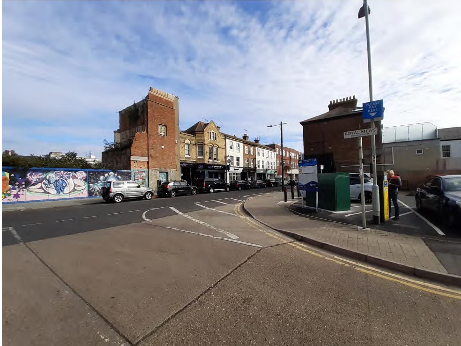
Neighbouring properties to the east of the site on Alexandra Street
