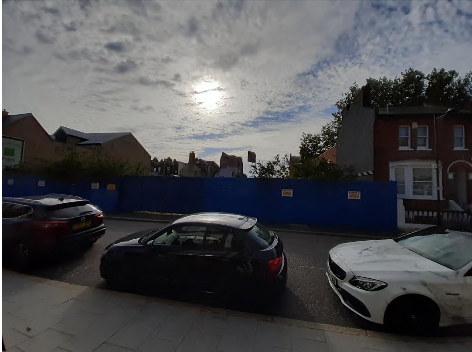
Clarence Street frontage of the site
